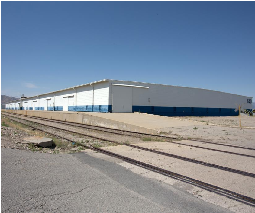
Former Army Depot Buildings
